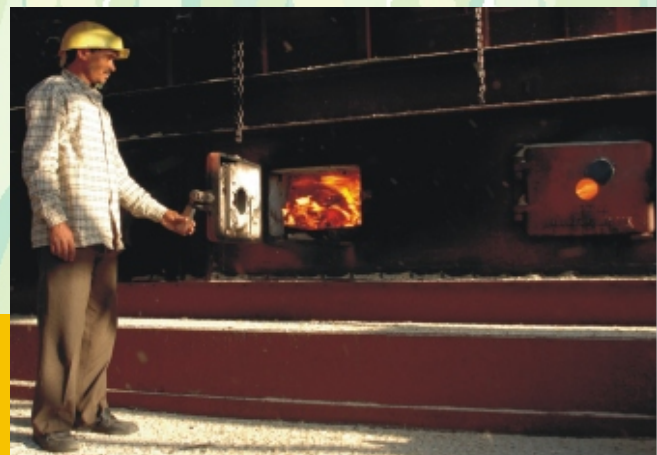
Bagasse, a by product of the sugar manufacturing process is used to generate power for captive consumption and export.
